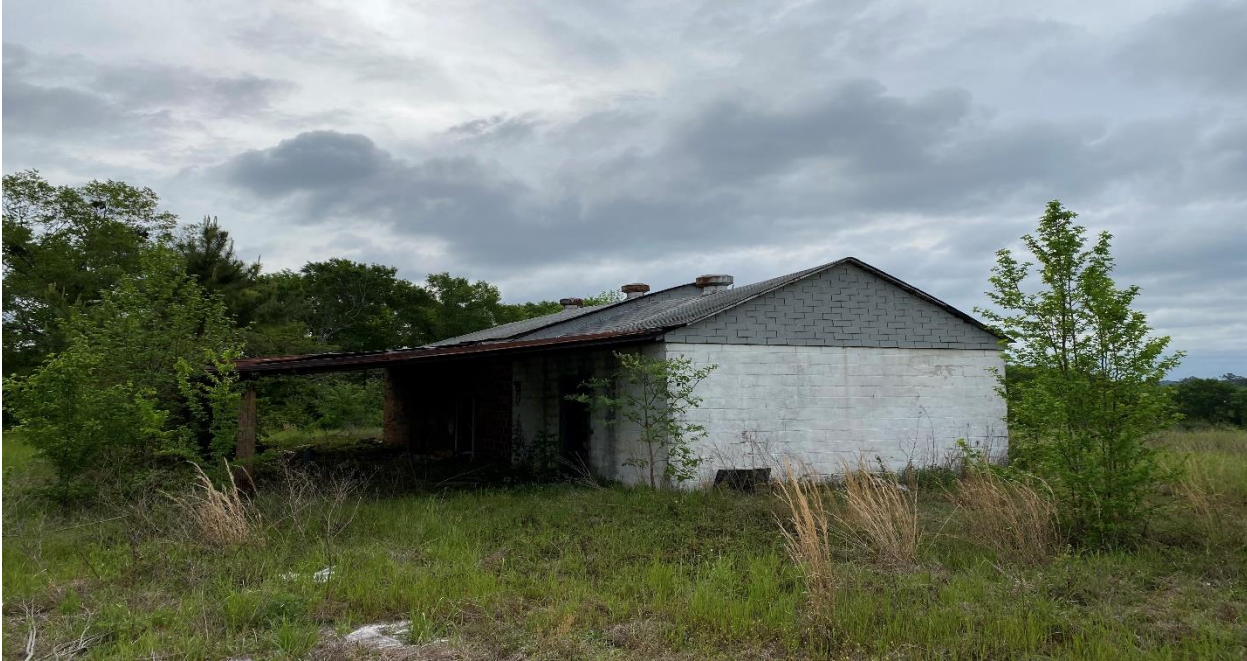
General Photo of Bldg. 1
